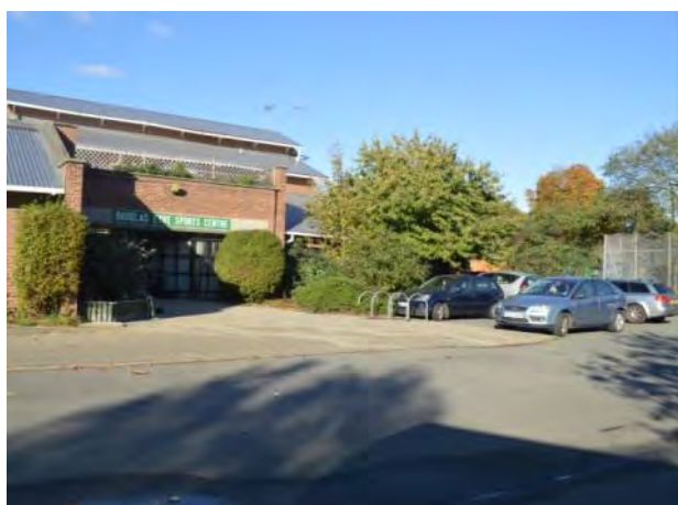
View of the sports centre building.
